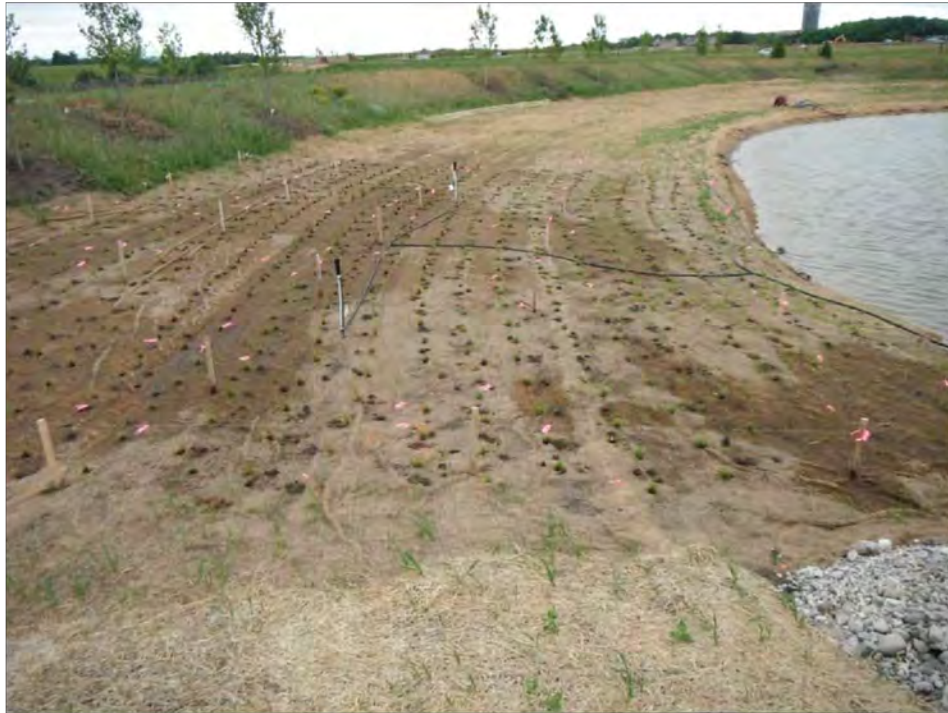
Photograph No. 1. Basin #1 Plug installation area.
