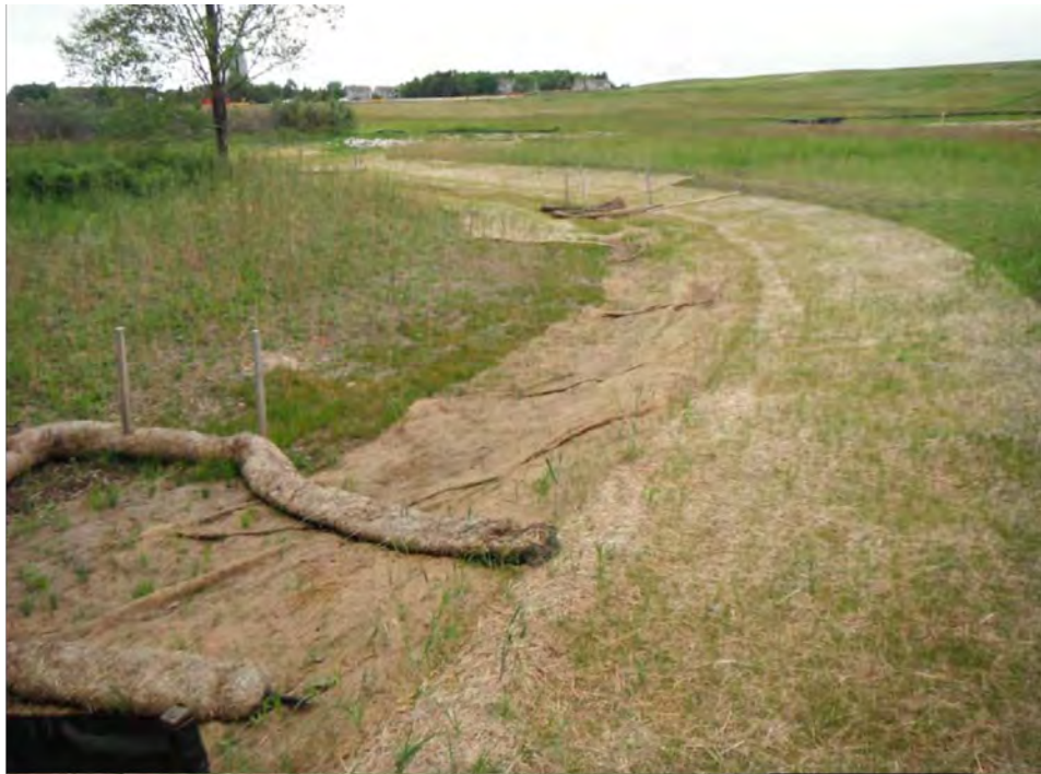
Photograph No. 19. Basin #2. Discharge swale to stream.
