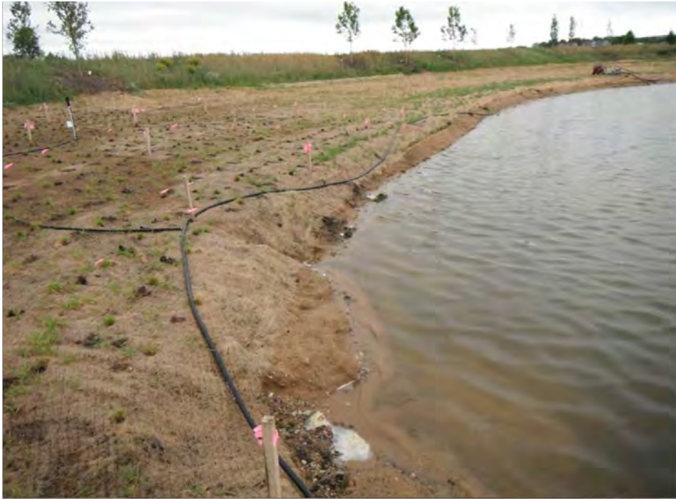
Photograph No. 2. Water level in Basin #1 below planting elevation.
