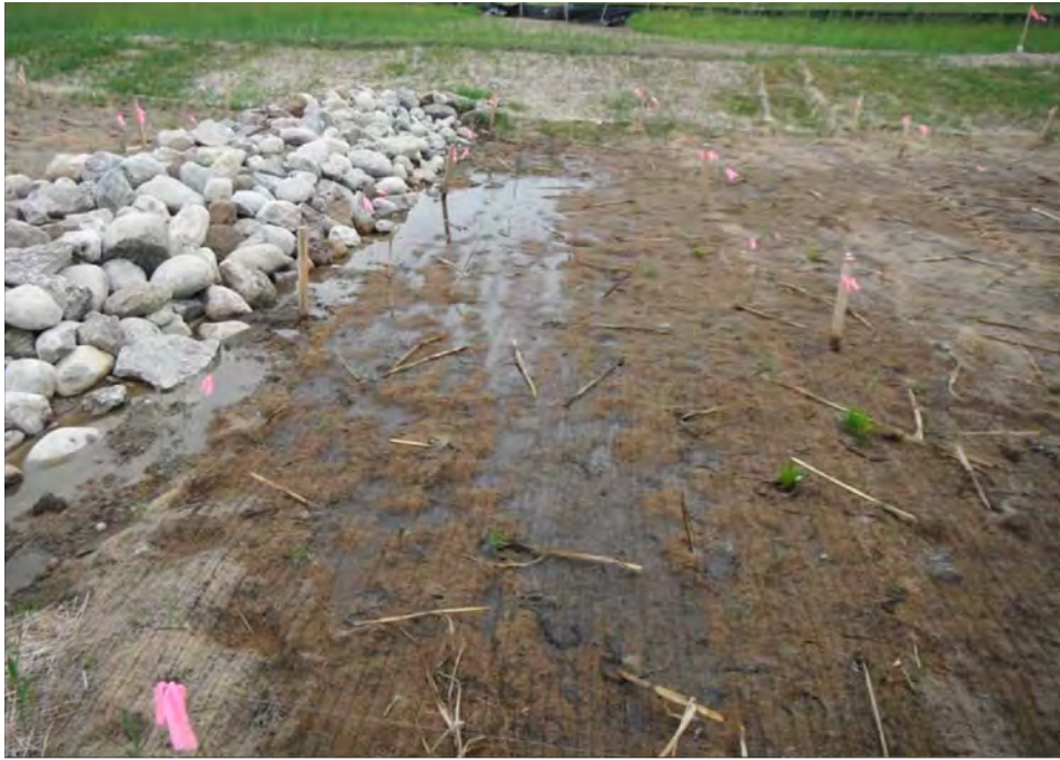
Photograph No. 15. Basin #2A. Inundation.
