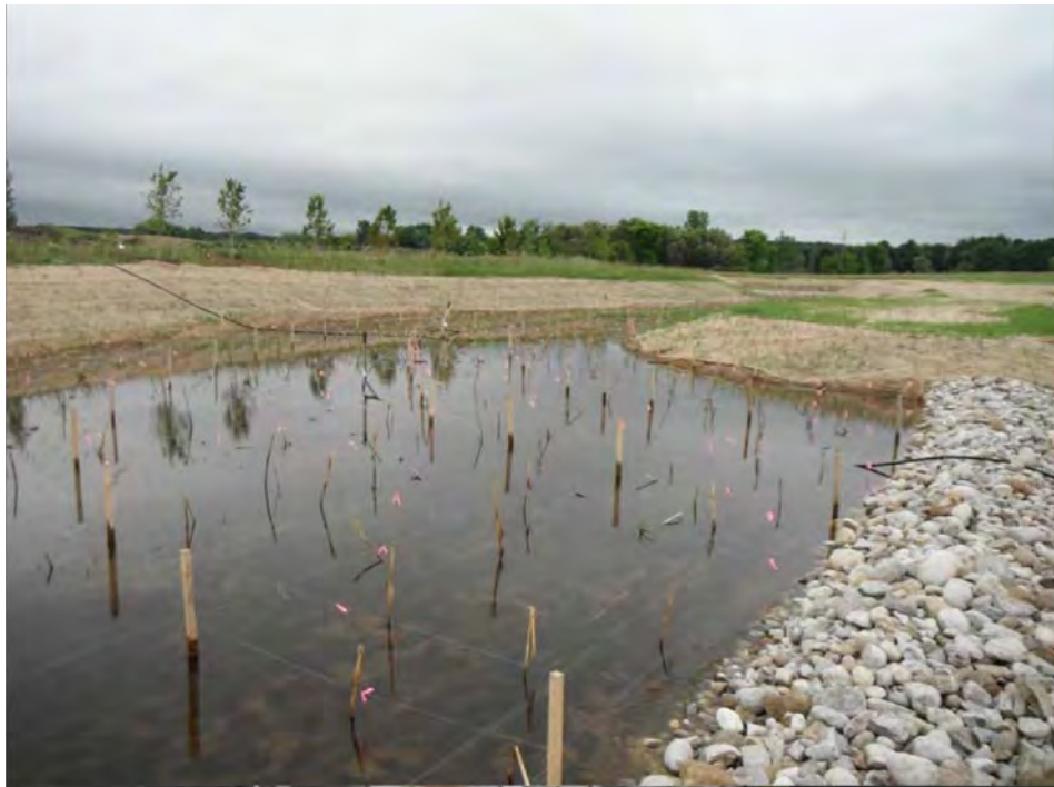
Photograph No. 4. Basin #1B
