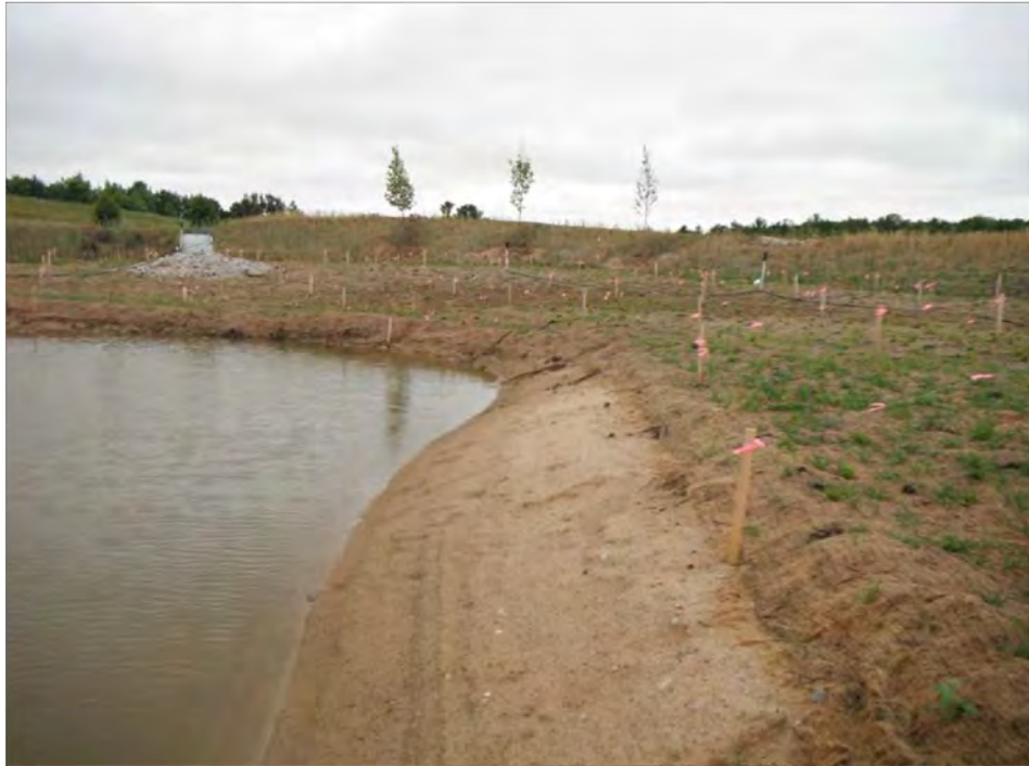
Photograph No. 9. Basin #2. Water level below planting elevation.
