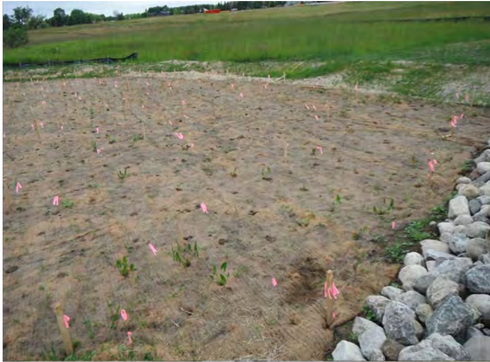
Photograph No. 17. Basin #2B. Facing NW.
