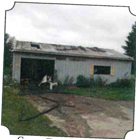
Garage Fire on Keystone Rd
