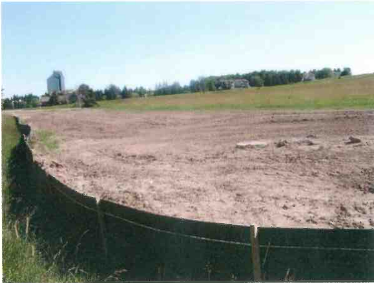
Photograph #20: Sediment build-up at silt fence at western boundary of the GTTC property, looking north. Taken by C. Grobbel, Grobbel Environmental & Planning, July 4, 2014.
