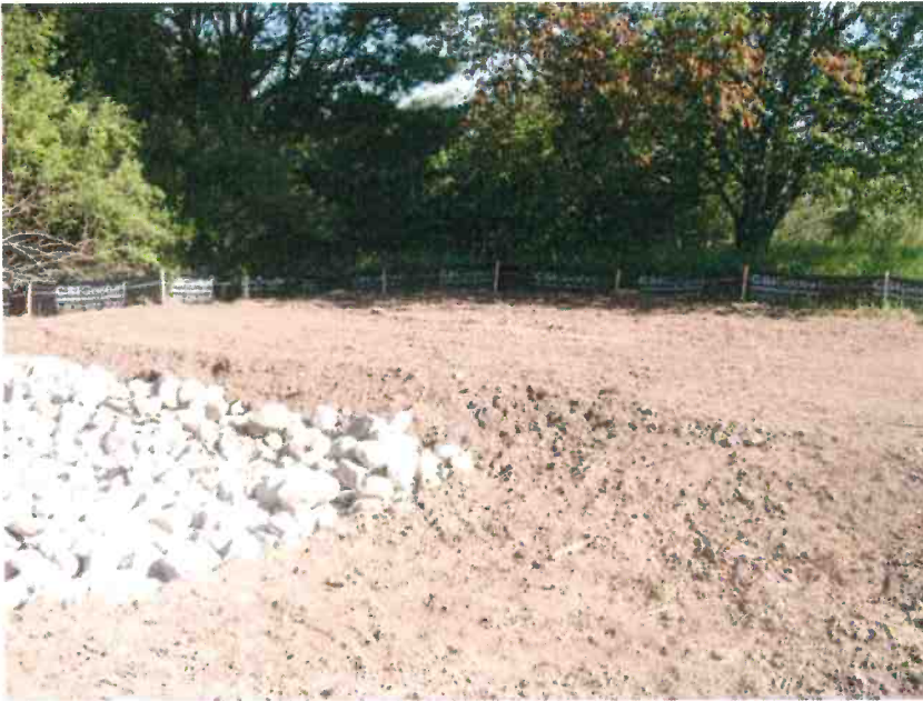
Photograph #10: South-central portion of the GTTC property looking north-westerly at the terminus of the grassed waterway. Taken by C. Grobbel, Grobbel Environmental & Planning, July 4, 2014.
