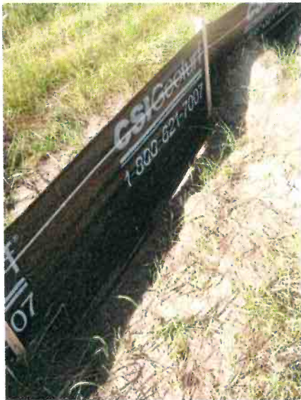
Photograph #1: Eastern portion of the GTTC property, showing improper installation of silt fence. Taken by C. Grobbel, Grobbel Environmental & Planning, July 4, 2014.
