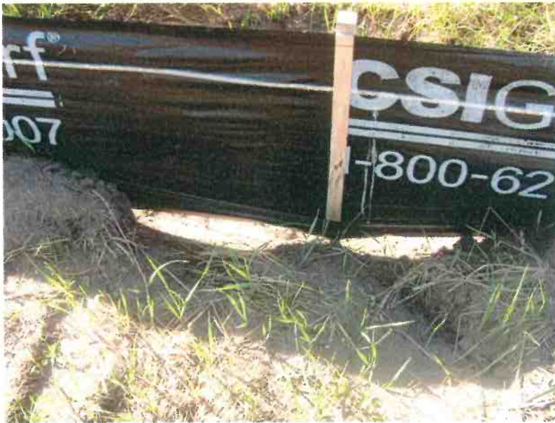
Photograph #2: Eastern portion of the GTTC property, showing improper installation of silt fence. Taken by C. Grobbel, Grobbel Environmental & Planning, July 4, 2014.
