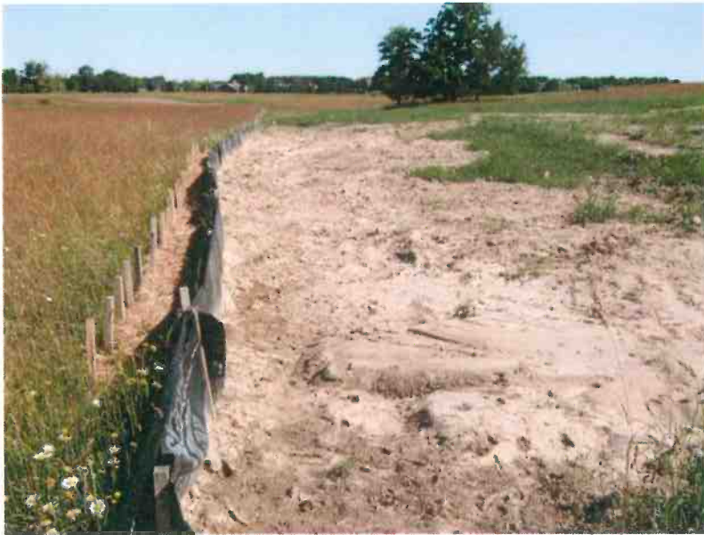
Photograph #16: Southwest corner of the GTTC property looking northerly at showing sediment/ponded area along silt fence. Taken by C. Grobbel, Grobbel Environmental & Planning, July 4, 2014.
