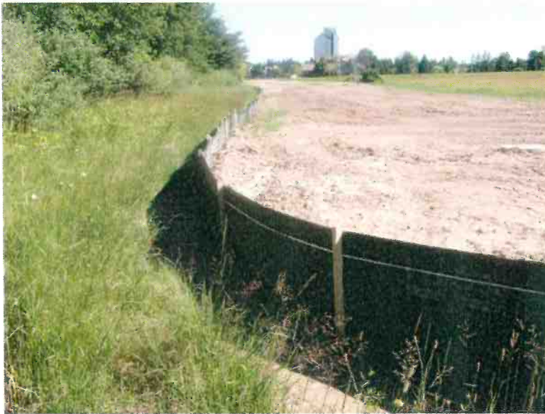
Photograph #19: Sediment build-up at silt fence at western boundary of the GTTC property, looking north. Taken by C. Grobbel, Grobbel Environmental & Planning, July 4, 2014.
