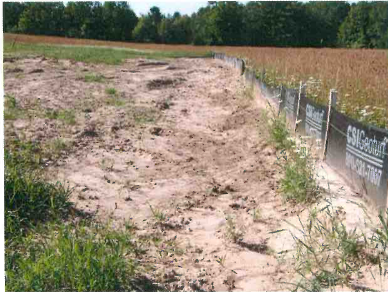
Photograph #17: Southwest corner of the GTTC property looking southerly at showing sediment/ponded area along silt fence. Taken by C. Grobbel, Grobbel Environmental & Planning, July 4, 2014.
