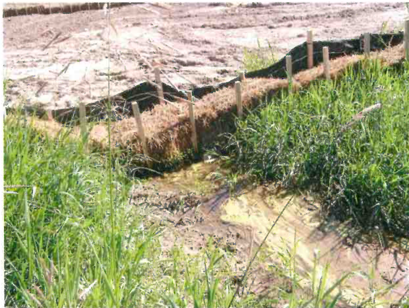
Photograph #15: South-central portion of the GTTC property showing sediment beyond silt fence/straw bale structure at the base of the swale. Taken by C. Grobbel, Grobbel Environmental & Planning, July 4, 2014.
