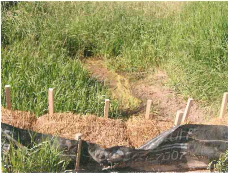
Photograph #14: South-central portion of the GTTC property showing sediment beyond silt fence/straw bale structure at the base of the swale. Taken by C. Grobbel, Grobbel Environmental & Planning, July 4, 2014.
