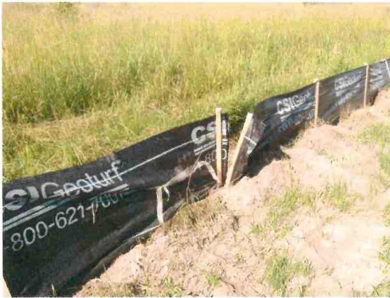
Photograph #4: Eastern portion of the GTTC property, showing improperly connected silt fence sections. Taken by C. Grobbel, Grobbel Environmental & Planning, July 4, 2014.
